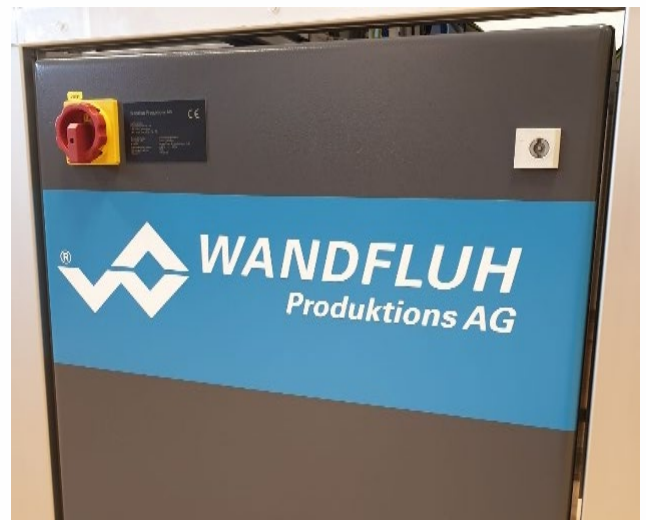
Wapro control cabinet construction
